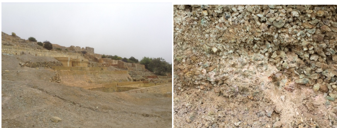
Figure 4.10: Left: General view of the condition of the La Cobaltera Plant: Right: Leach pad gravels from the La Cobaltera plant. The photo shows erythrite precipitates, copper sulfates and gypsum.
